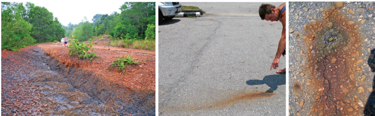
Figure 3. Damage to road infrastructures by erosion and corrosion of concrete and road material (pH 3.5 - 4.2) from the exposure (oxidation) of pyrite contained in the pyrite-rich shale at Tungku.
